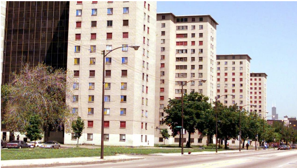
THE ROBERT TAYLOR HOMES, SHOWN FRIDAY, MAY 28, 1999, ARE ONE OF THE PUBLIC HOUSING DEVELOPMENTS THAT WILL ONCE AGAIN COME UNDER CONTROL OF THE CHICAGO HOUSING AUTHORITY. AFTER BEING TAKEN OVER BY THE U.S. DEPARTMENT OF HOUSING AND URBAN DEVELOPMENT IN 1995 FOLLOWING A SERIES OF CHAOS SCANDALS, HUD RETURNED CONTROL TO THE CITY THURSDAY. (AP PHOTO/CHARLIE BENNETT)
